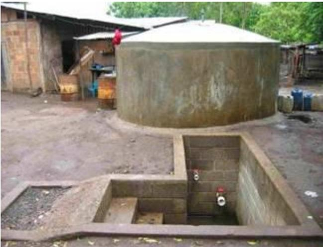
▲ A completed 27,000 litre water tank with domed roof and tap station. The smaller valve at a higher level draws water for domestic use. The larger valve at a lower level drains the tank completely for cleaning purposes.
