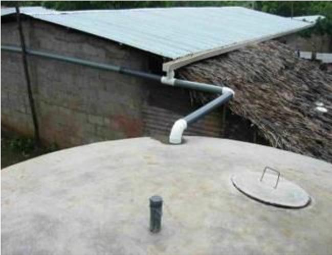
▲ Gutters from both sides of this corrugated iron roof channel rainwater into this 31,000 litre tank. The roof of the tank protects the water supply from contamination and prevents mosquitoes from breeding.
