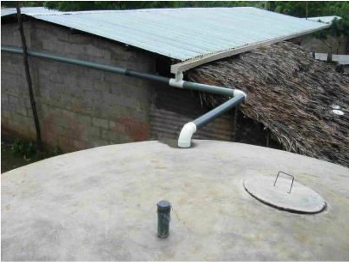
▲ Gutters from both sides of this corrugated iron roof channel rainwater into this 31,000 litre tank. The roof of the tank protects the water supply from contamination and prevents mosquitoes from breeding.
