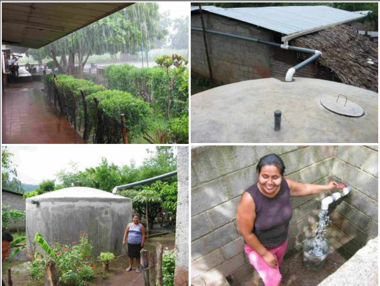
Rainwater harvesting from the pilot project at San Jacinto in 2005 (clockwise from top left): plentiful rain falls during the wet season; rainwater harvested from roofs is collected in large tanks; this tank can store enough water to last through the dry season; at last, Luvy Vallejos has water at her own home!
